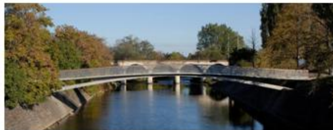
Fig2 Stress Ribbon Bridge Supported On Arches
