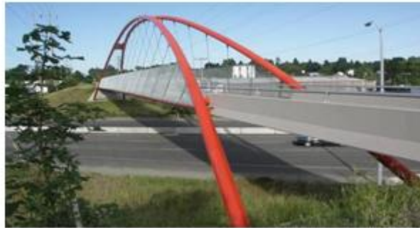
Fig.3 Stress Ribbon Bridge Suspended On Arches
