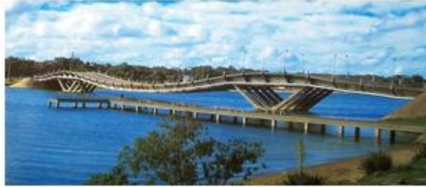
Fig 1 Stress Ribbon Bridge
